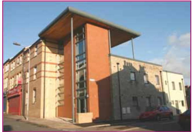
Tapscott House, Vere Street, Barry, Vale of Glamorgan
